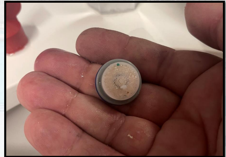
Faucet aerator with negligible debris
