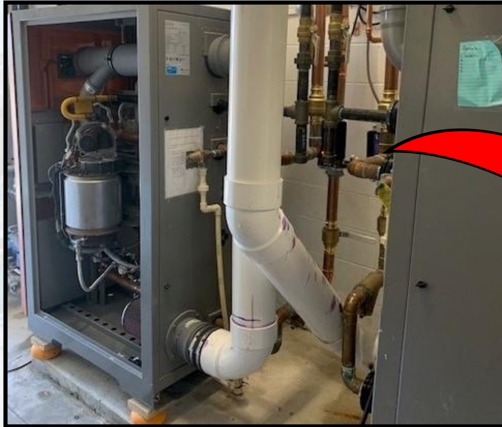
Tankless water heaters and HydroFLOW devices
