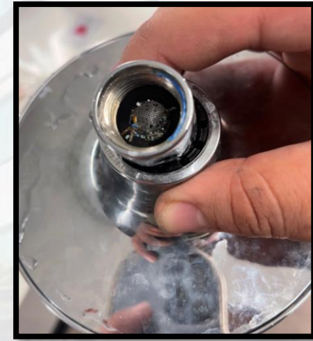
Showerhead with a little debris
