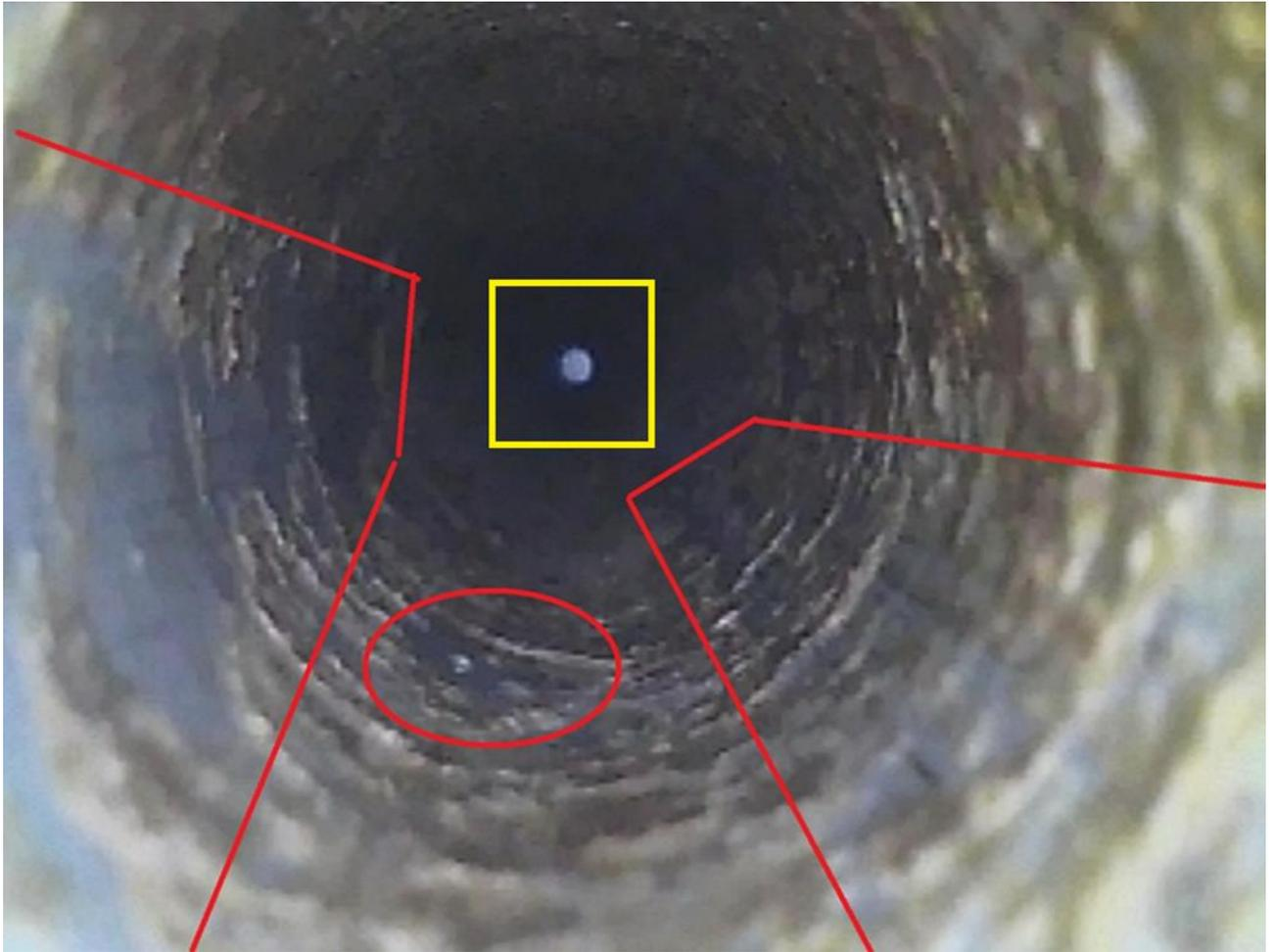
*Removing the carbonate layer from the wall of the heat transfer tube using metal brush. Red sectors - zones of removed sediments, yellow sector - clean section at the end of the tube.*
