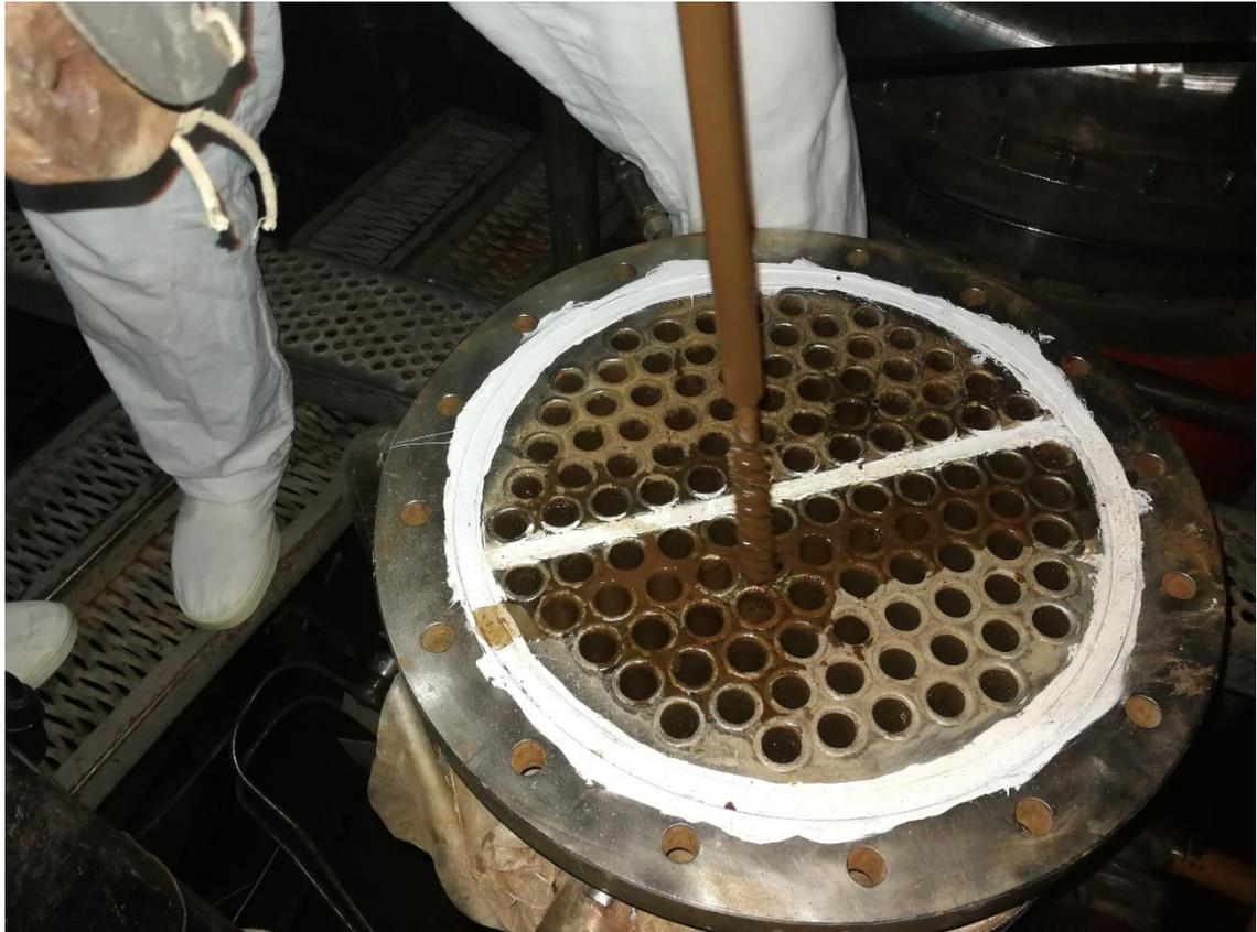
*Cleaning the heat exchanger tubes with a steel wool*
