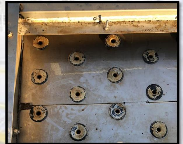
Limescale on cooling tower nozzles
